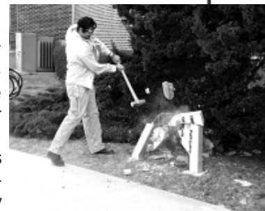
Design Week 1999 - Architecture Day: Concrete demolition event
